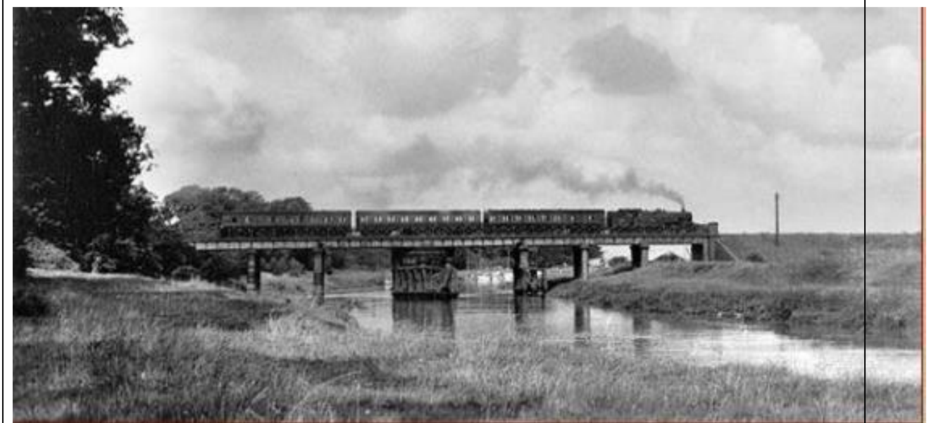
The River Douglas bridge looking north in August 1964 as a Preston-bound train crosses over. In the middle of the river the section on which the bridge had swung can be seen. It had however been fixed into position since 1913.
