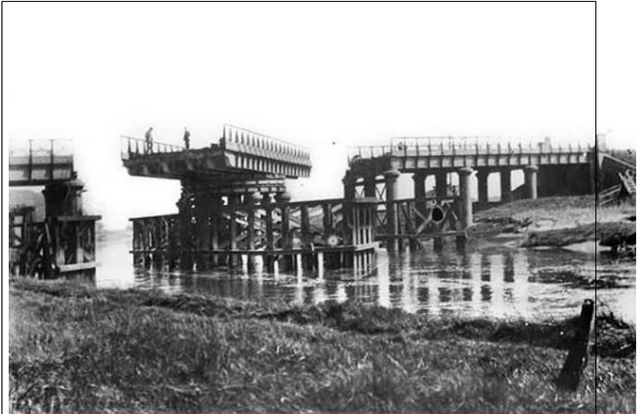
A picture from the early 20th Century shows the River Douglas Bridge in the open position.
